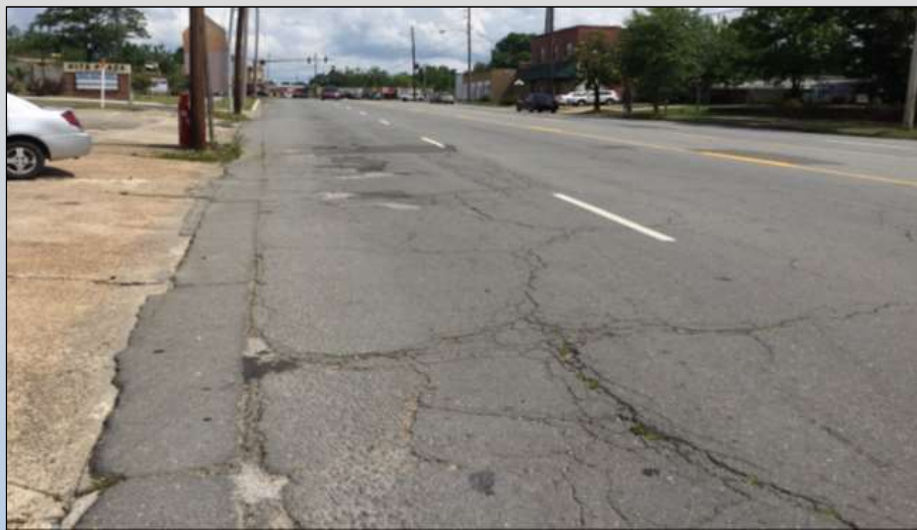
Garland County Highway 270, Section 6 Log mile 0.0 - 2.0 just east of Highway 7 on MLK Expressway
